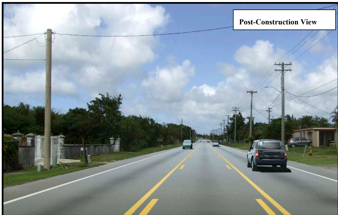
Figure 15.2-1. Key Viewpoint 1: GRN #57, Route 28 Widening
