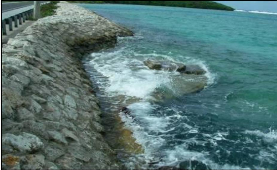
**Figure 4.1-34. Coastal Erosion Protection along Route 11**
