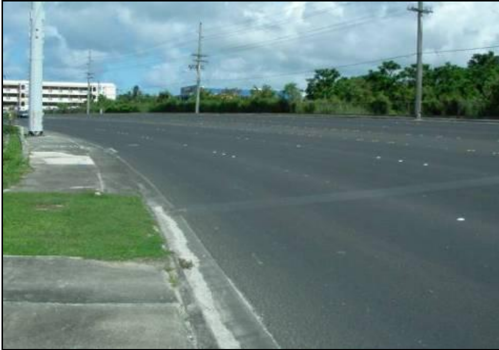
Figure 4.1-17. Route 16 – Curb Outlet at Low Point to Sink
