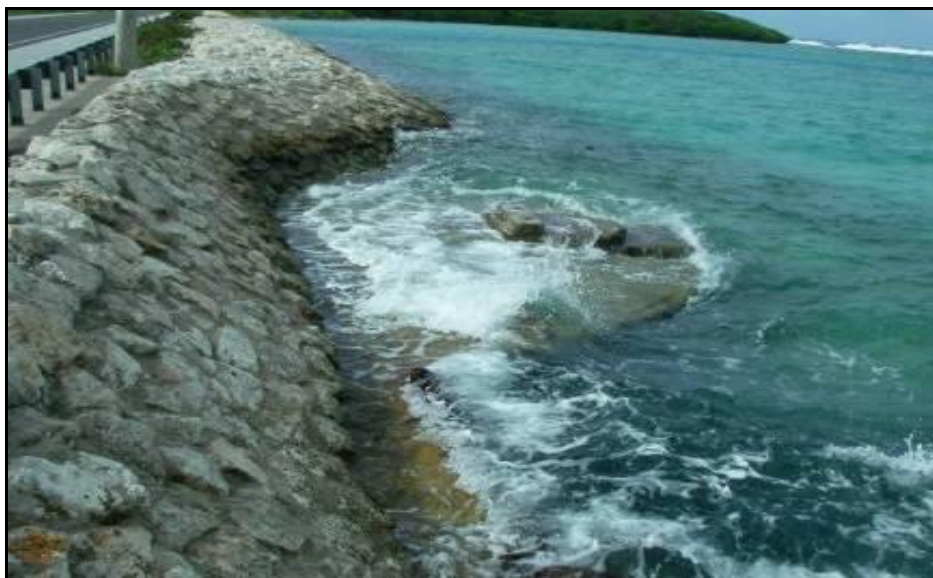
Figure 4.1-34. Coastal Erosion Protection along Route 11
