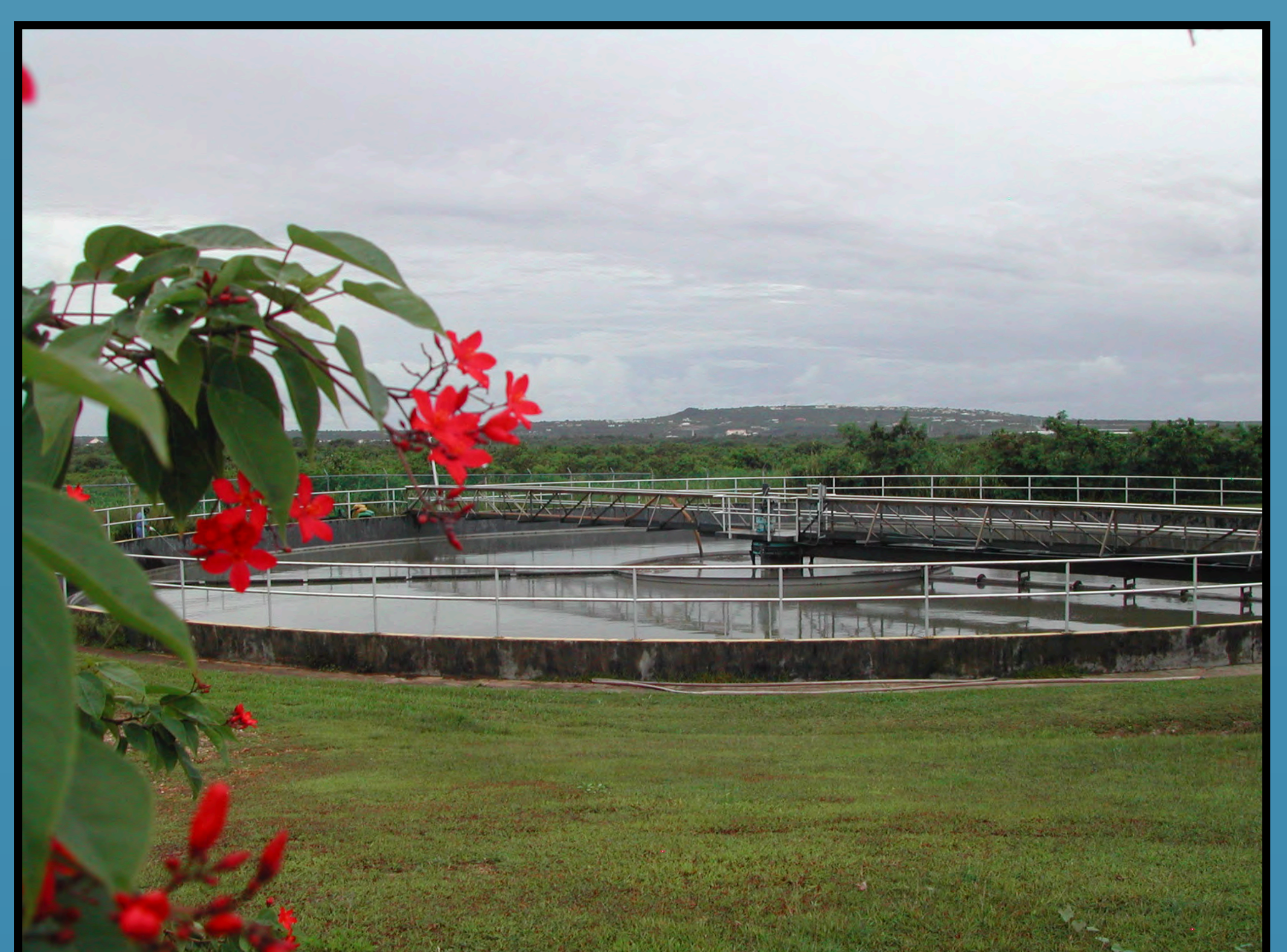
Northern District Wastewater Treatment Plant
